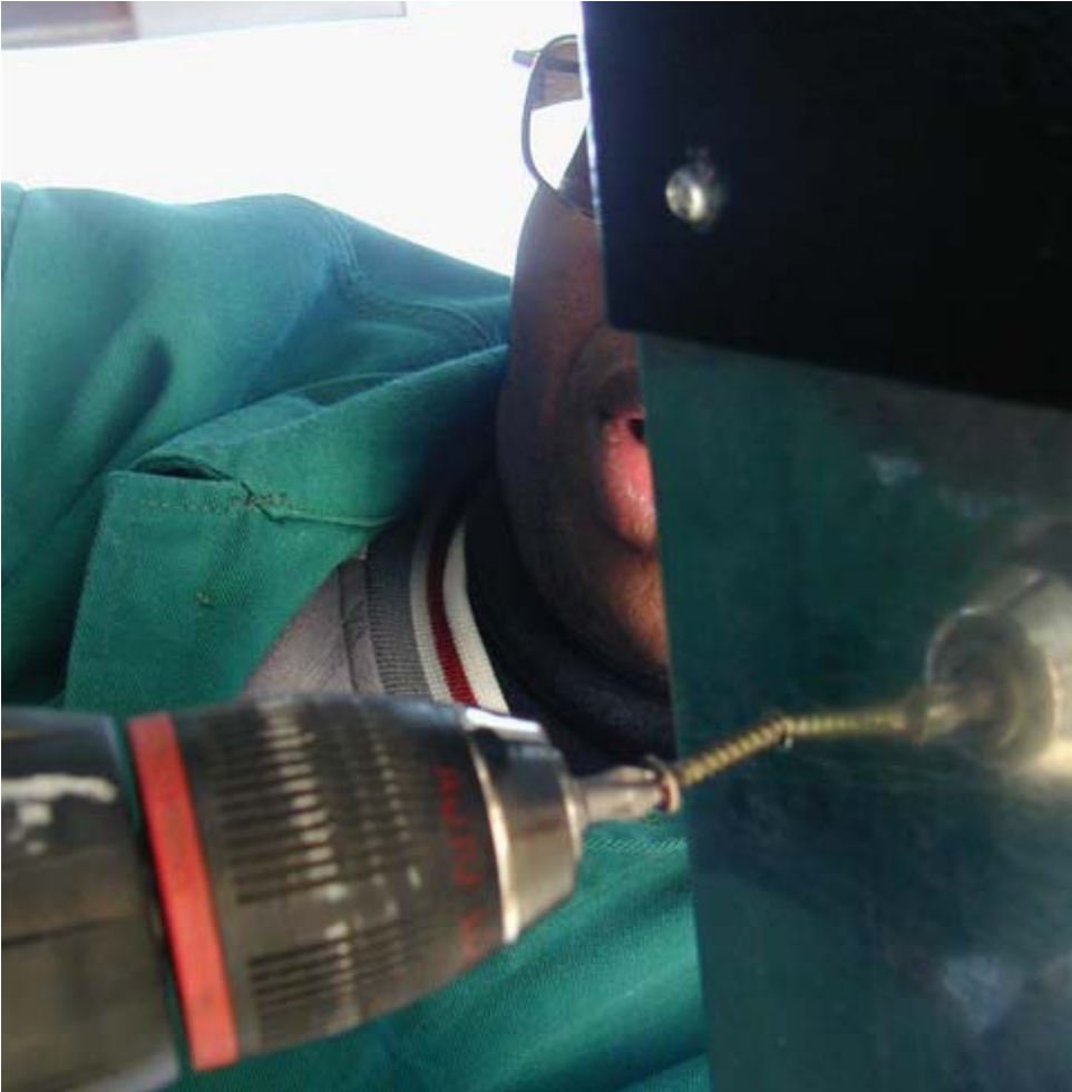
Fig: 26 screw wooden floor from underside
