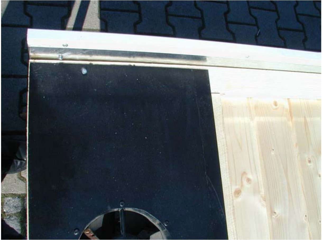
Fig: 31 make holes and screw on the fan plate
