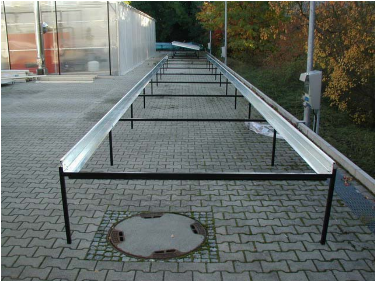
Fig: 20 finished base frame with u-profile
