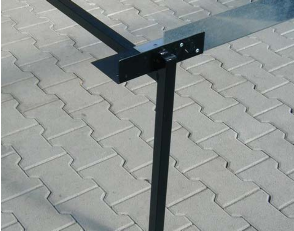
Fig: 9 base frame assembling
