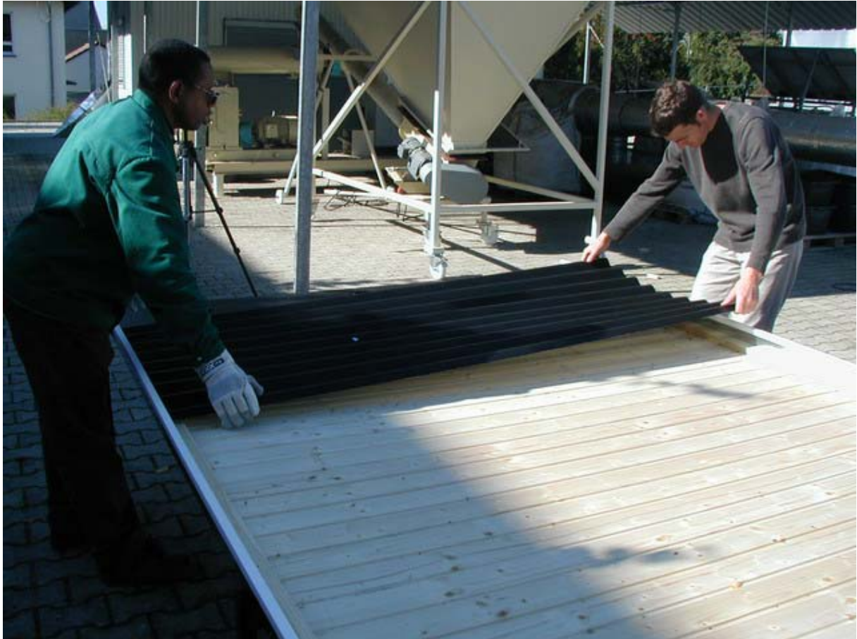
Fig: 35 insert the corrugated iron
