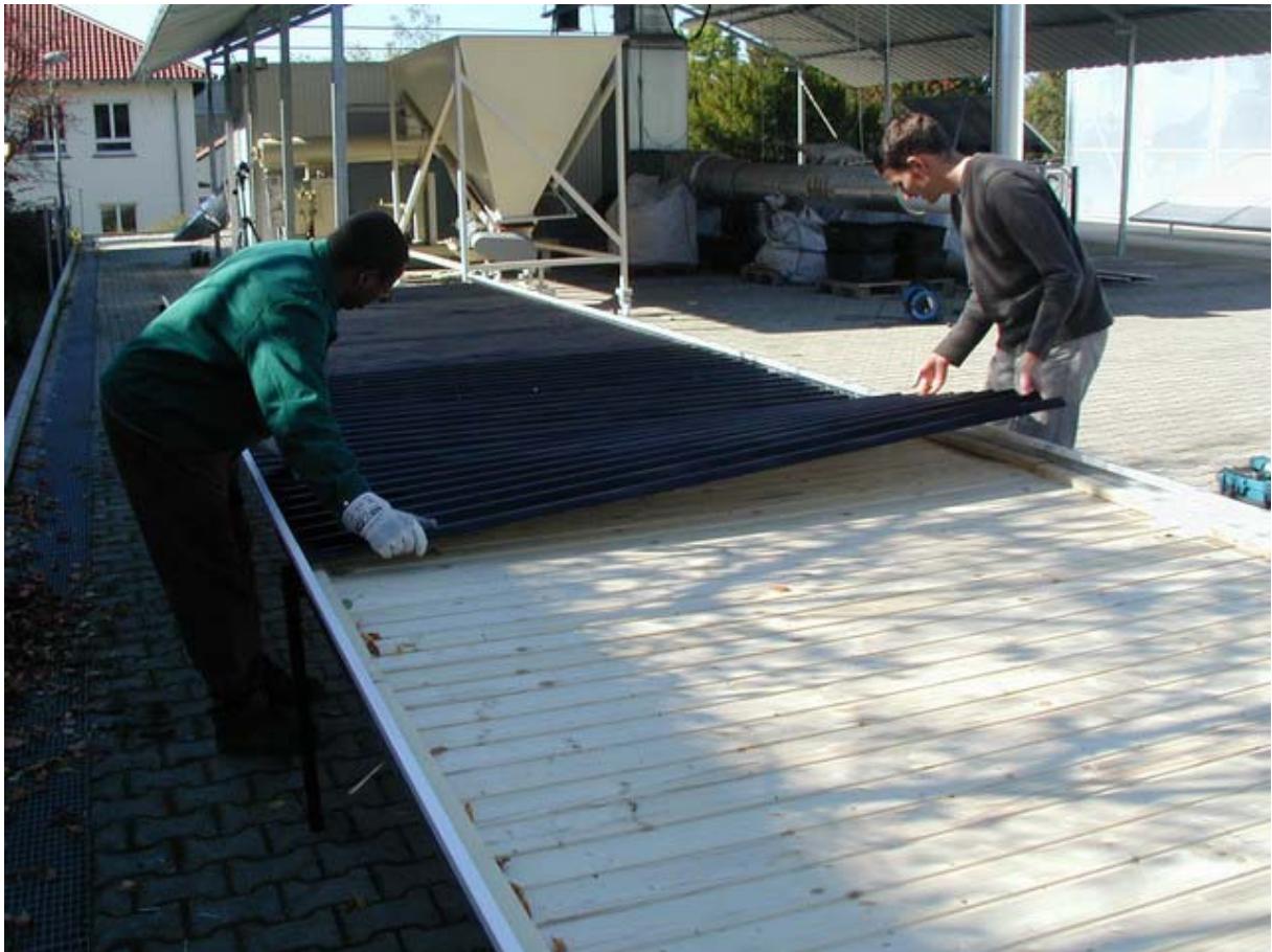
Fig: 37 insert the corrugated iron
