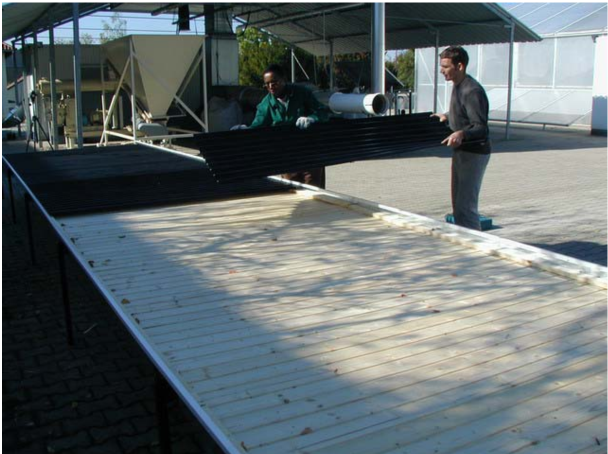
Fig: 36 insert the corrugated iron
