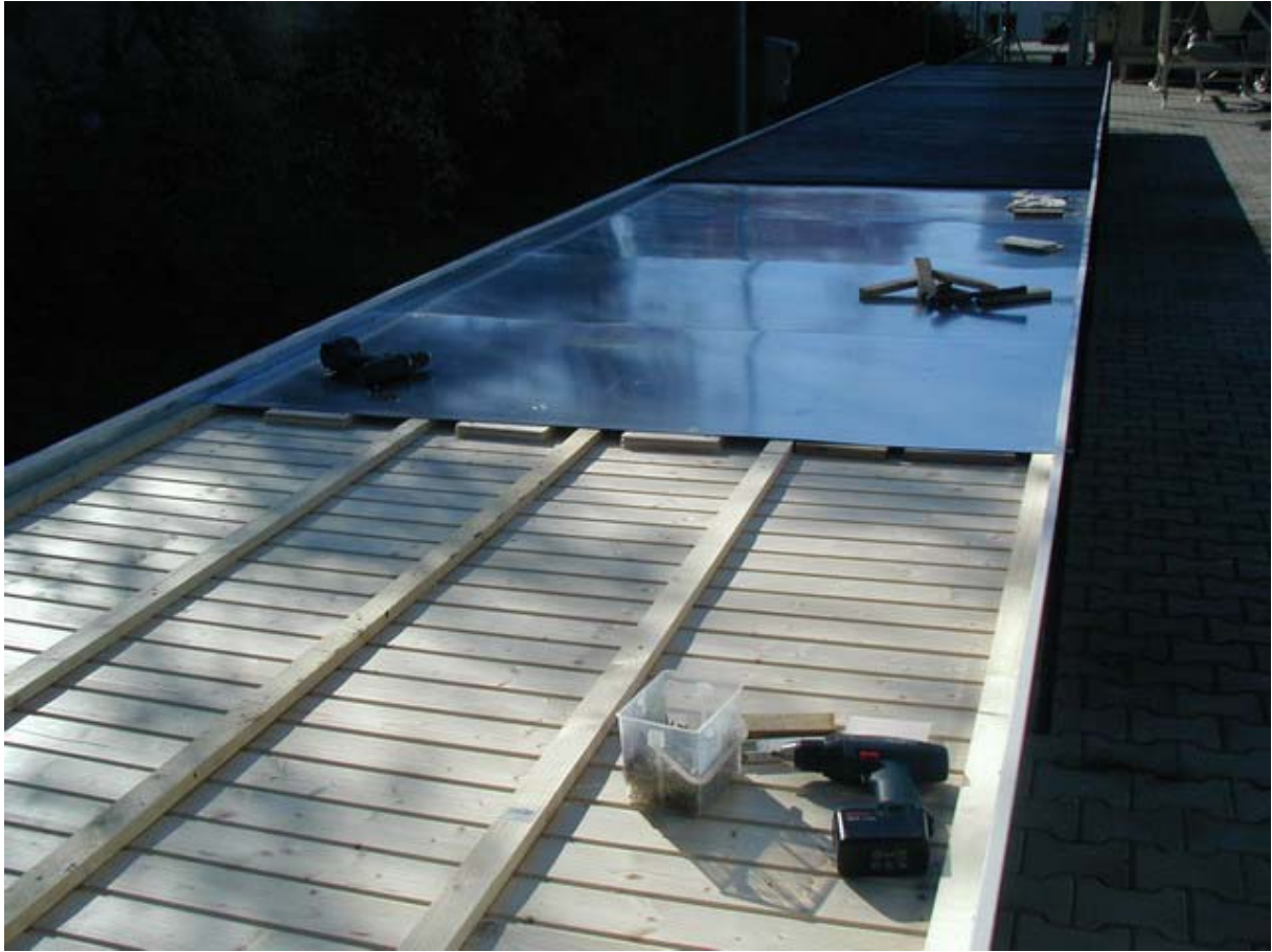
Fig: 42 insert the blank sheet
