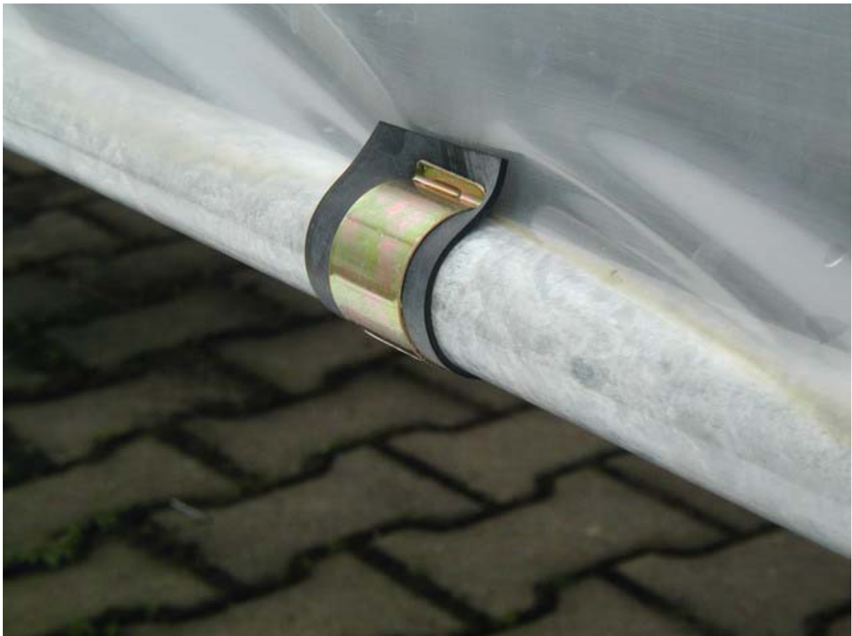
Fig: 56 foil clip with a rubber layer to protect foil
