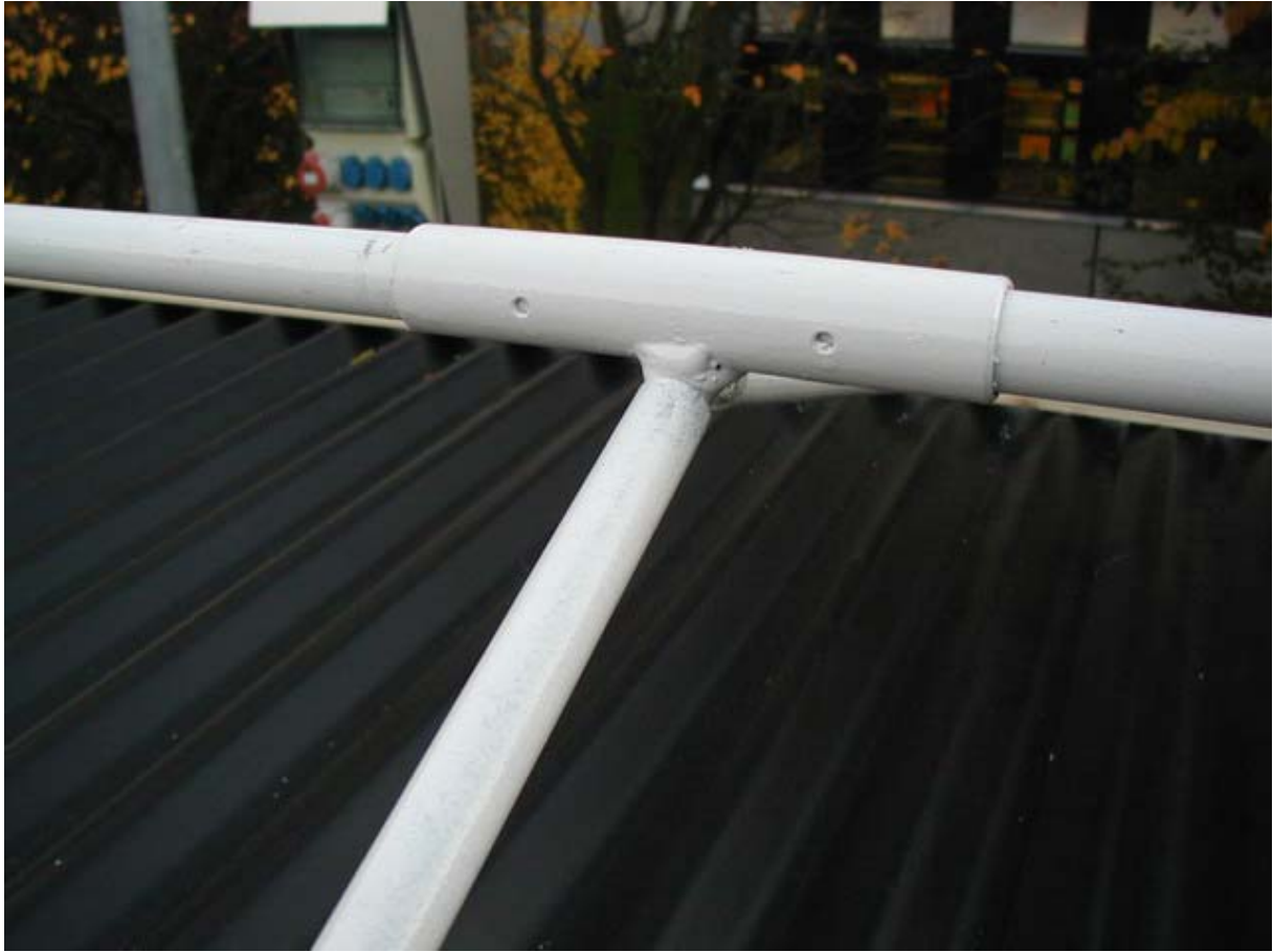
Fig: 47 roof connector assembled with roof rack and roof pipe
