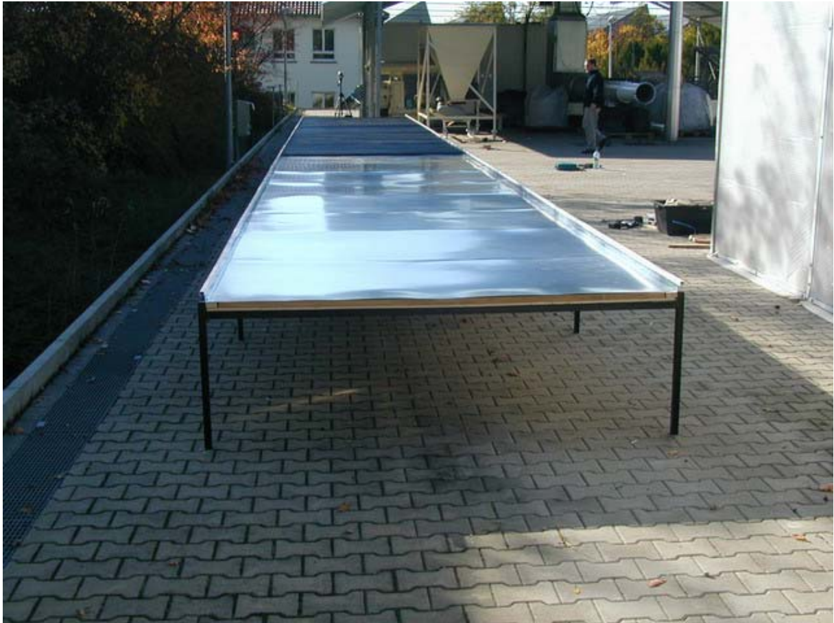
Fig: 44 finished base frame with absorber and drying area
