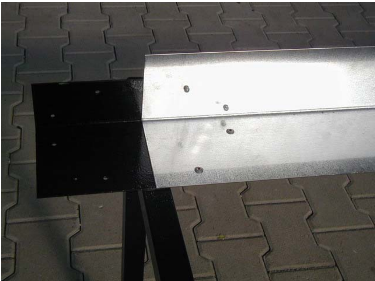
Fig: 10 base frame assembling
