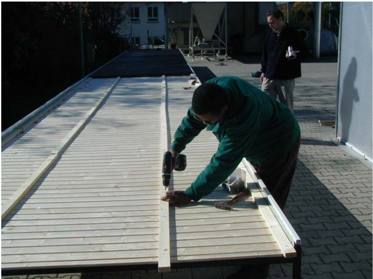
Fig: 41 screw on wood strip to stabilize blank sheet
