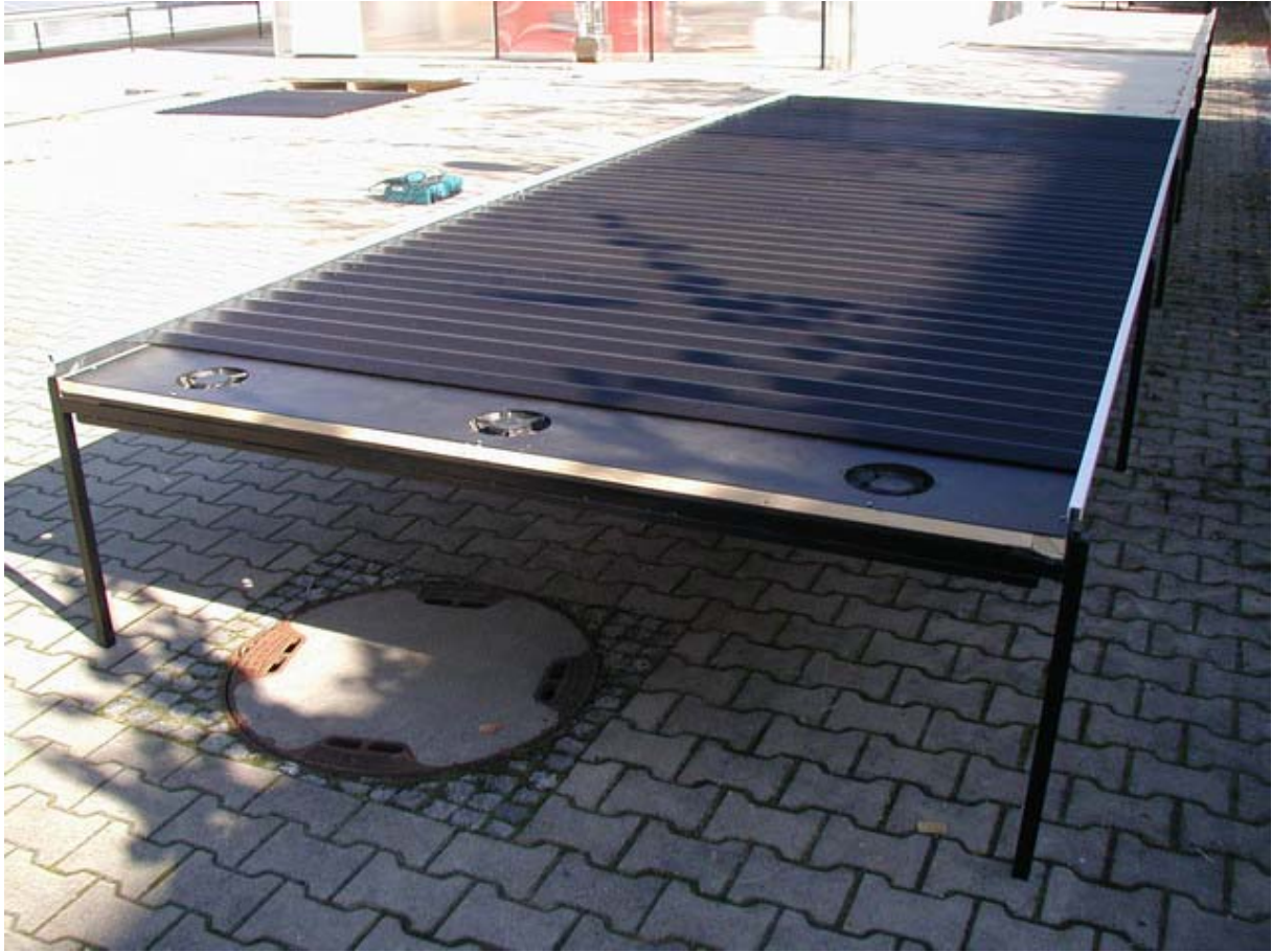
Fig: 39 make sideward holes and screw on the corrugated iron
