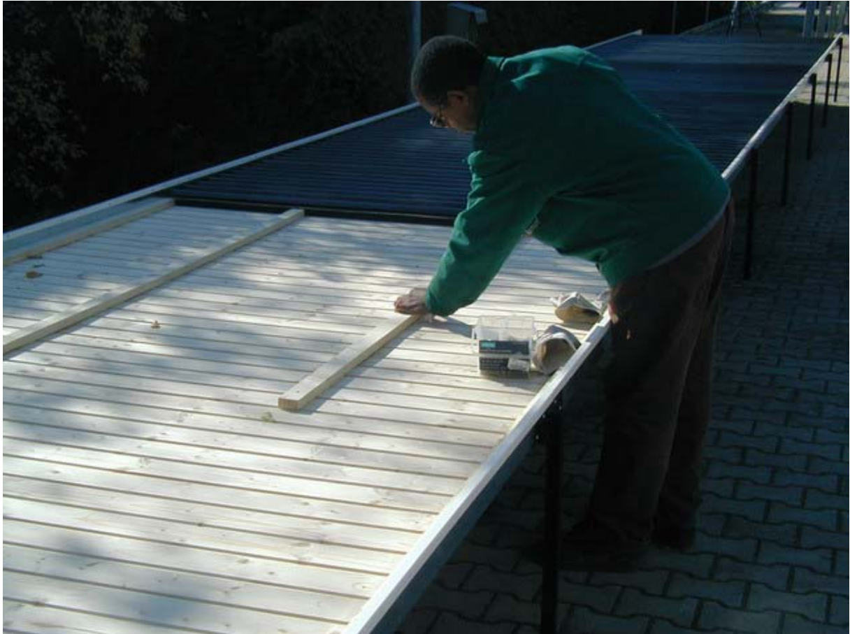
Fig: 40 screw on wood strip to stabilize blank sheet
