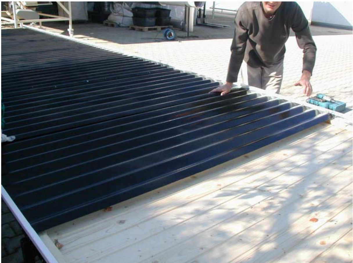
Fig: 38 insert the corrugated iron
