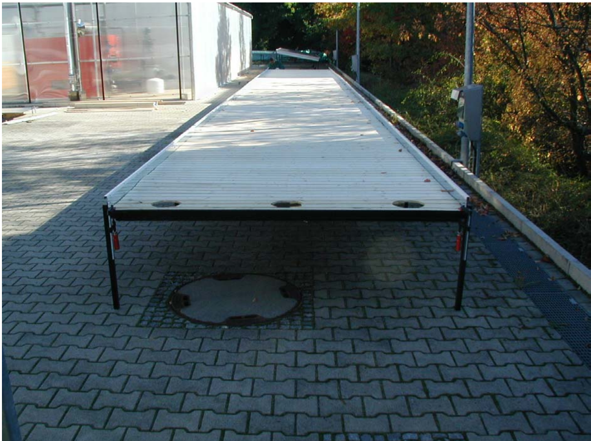
Fig: 24 finished wooden floor
