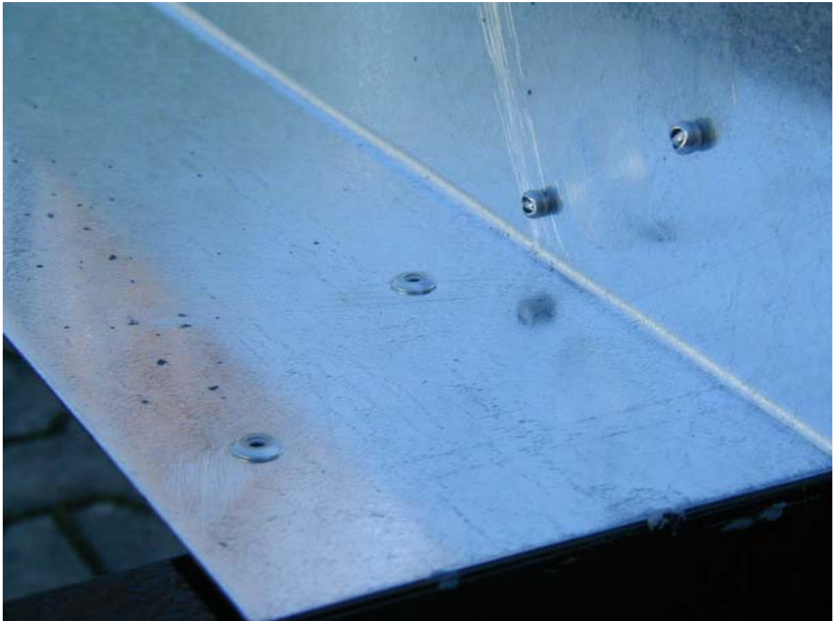
Fig: 8 finished rivet from inside
