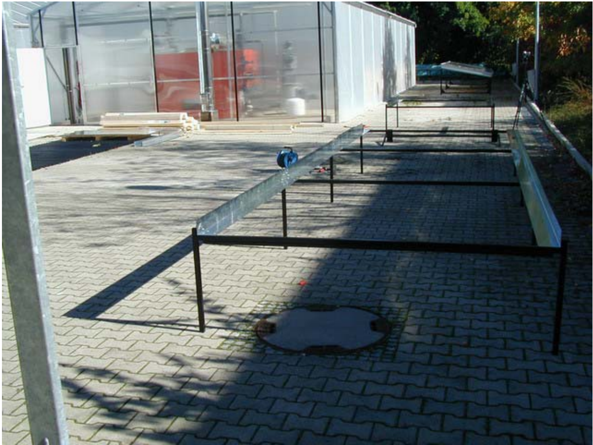
Fig: 15 base frame assembling short time before finished
